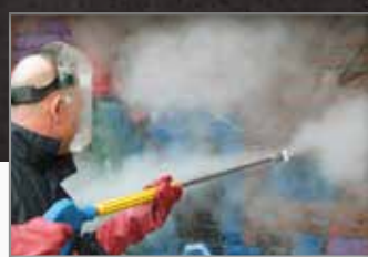
Graffiti removal: without chemicals
